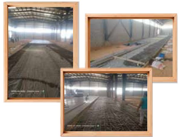
• Construction of factory floors and warehouses for Kernell Trade and Export Company Alef District - Fifth Settlement.
